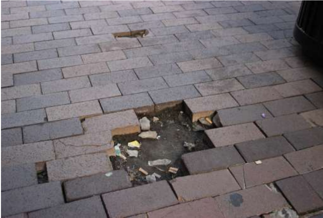
Image 4: Missing bricks pose safety risks near the Convention Center.
